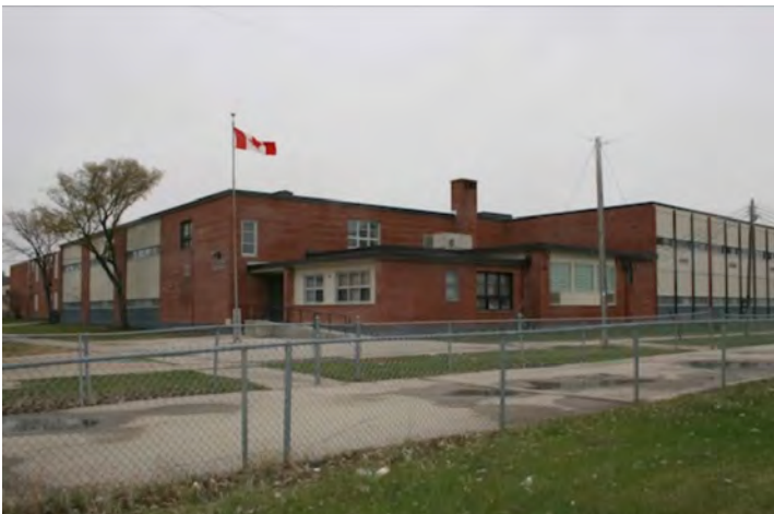
North-west facing corner, at the corner of Speers Rd. and Winakwa Rd. prior to Student Commons renovation (photo from Winnipeg Architecture Foundation https://winnipegarchitecture.ca/296-speers-road/ )
