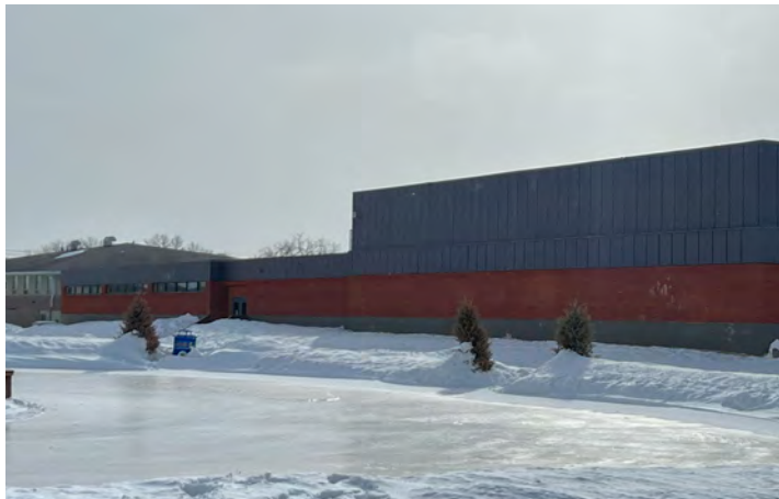
1969 Addition of gymnasium, library and practical arts
