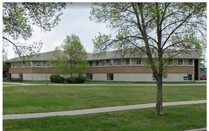
Current 2-storey classroom hexagon pod
