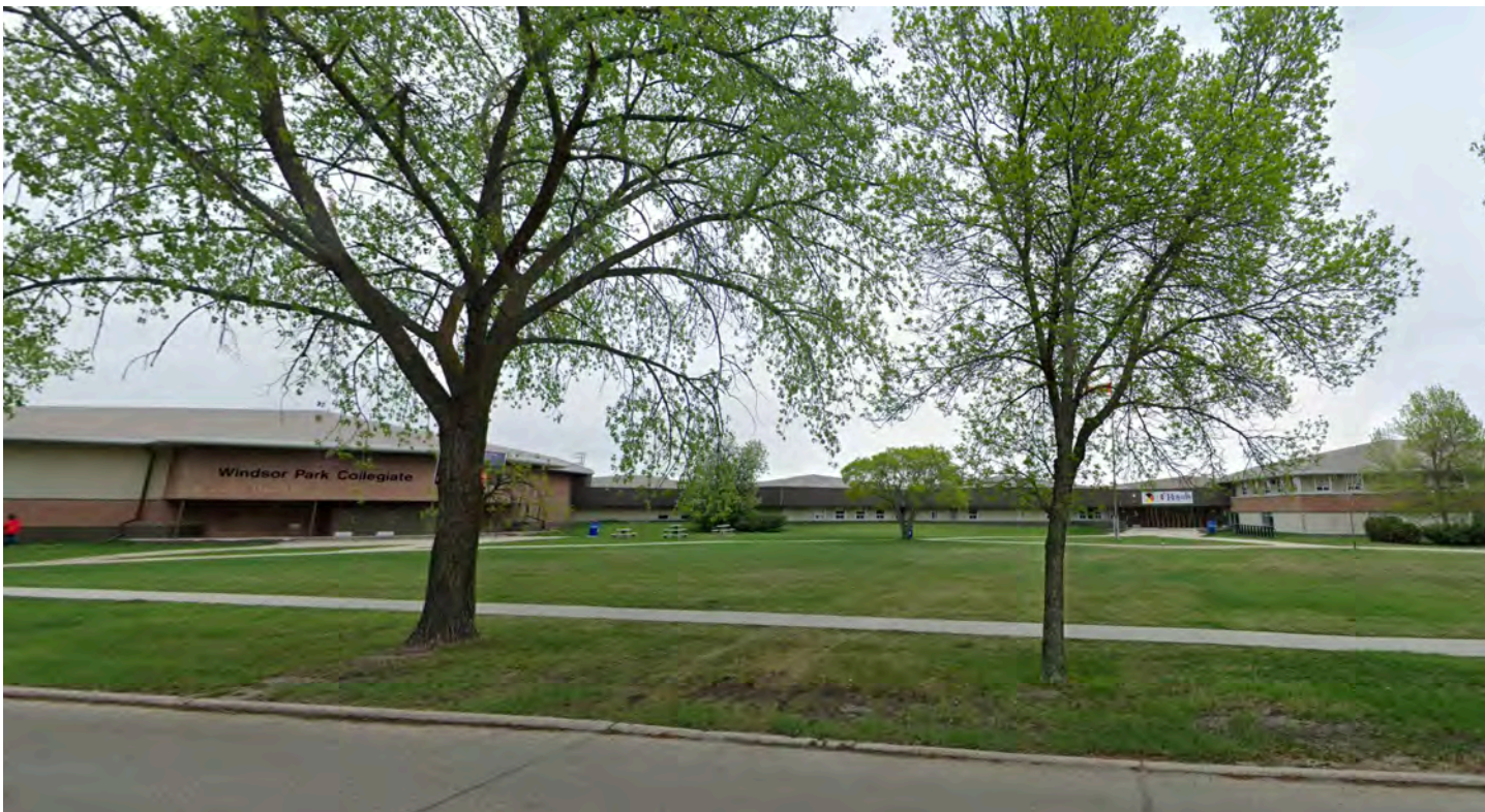
Front of school along Cottonwood Road, with gymnasium to the left; 2-storey classroom pod to the right, and central classroom and administration pods in the centre with main south entry
