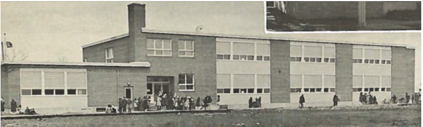
**Originally constructed building on the left (north), with two-storey addition in 1961 to the right (south)
