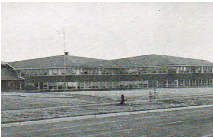
**Original construction - 2-storey classroom hexagon pods
