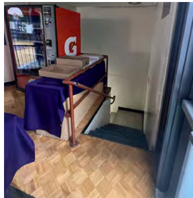
Stair to basement
