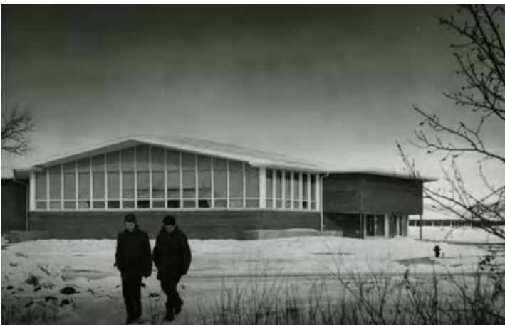
**Original construction - gymnasium, south facing
