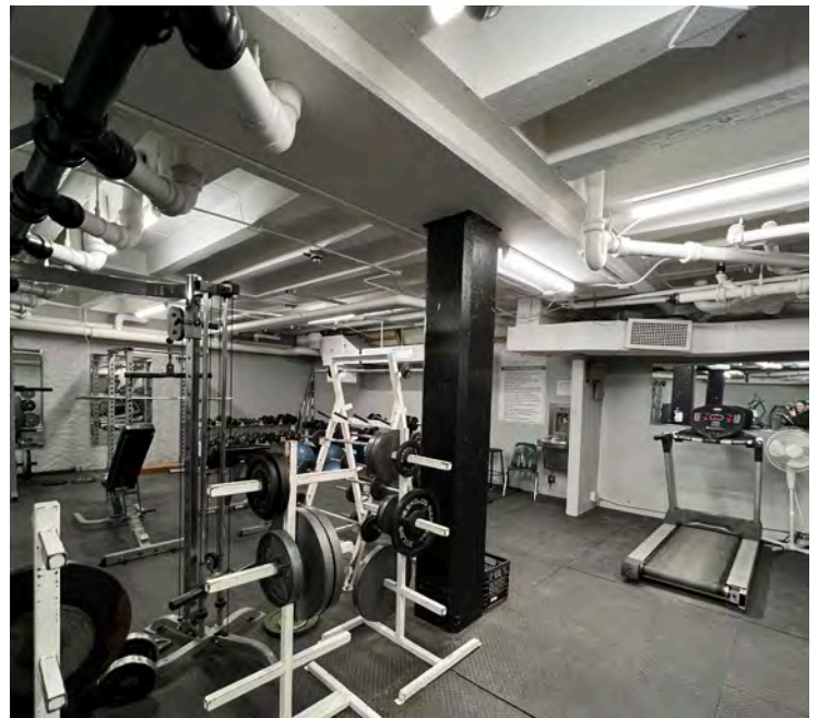
Fitness Room, exposed mechanical and electrical on concrete structure
