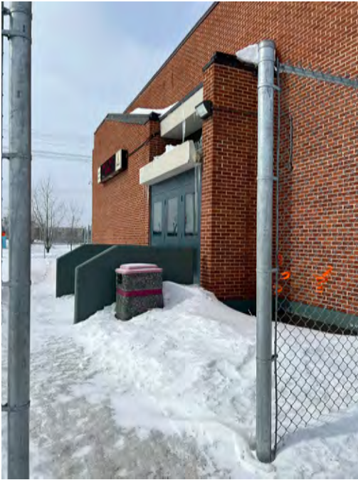
South exit from Gymnasium
