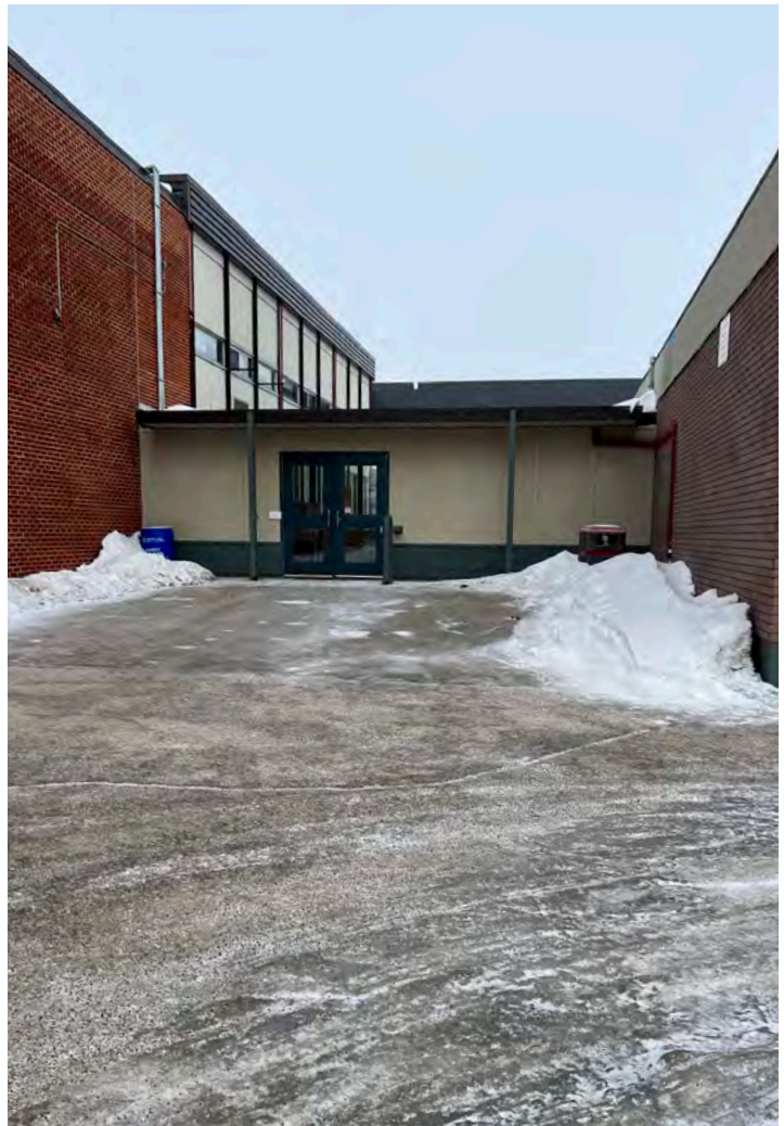
Main entrance accessed from south parking lot, into 1964 Addition "link".
