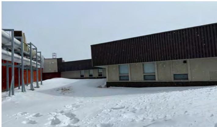
Link between original single-storey hexagon pod and 1969 addition (practical arts space)
