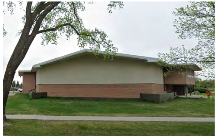
Current gymnasium, with original windows filled-in
